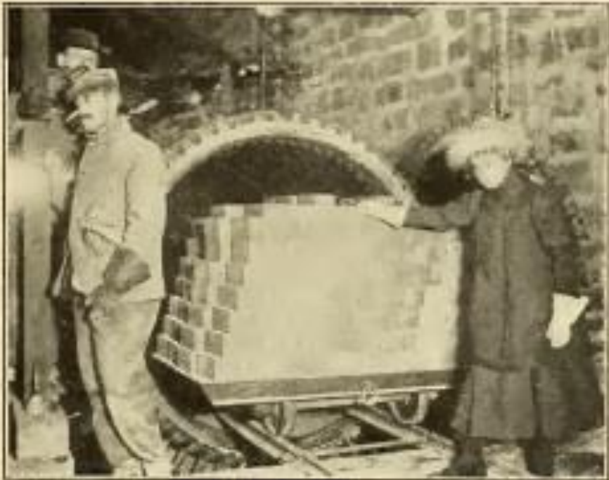
FIG. 12.—Hardening cylinder
